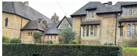
Preparations are underway at Mary's House.
